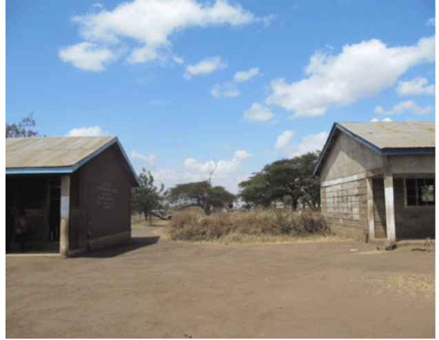
Matepes primary : a hole between 2 classrooms, waiting for well-wishers to build the missing class.
