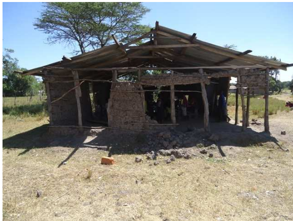
Inkorienito, in Transmara : Ruines of nursery class after downpour, last year. Probably demolished because dangerous to collapse.
