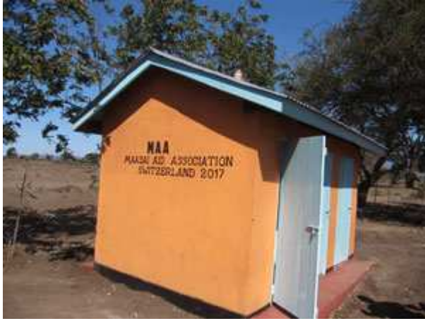
The 6 new sanitaries necessary with the school extension at Matepes primary
