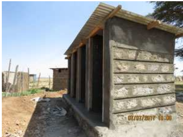
The 4 new sanitary (without doors here, as they get still dry) which were necessary with one more class room.
